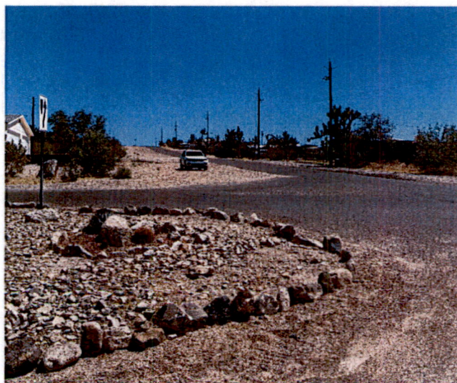
Figure 3: The Perspective of a Westbound Driver Ensuring there are no Oncoming Northbound Vehicles on Sandy Point Drive
