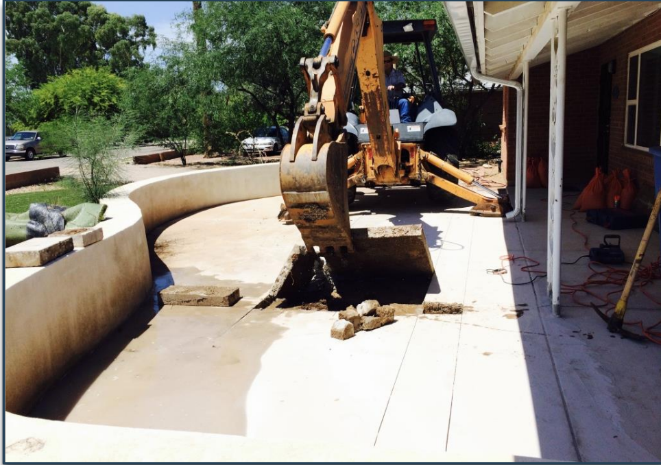
Photograph 7-4 The hardscape receiving roof runoff from downspouts that drained toward the foundation was removed and replaced with rain gardens and swales. Photo courtesy of Watershed Management Group.
