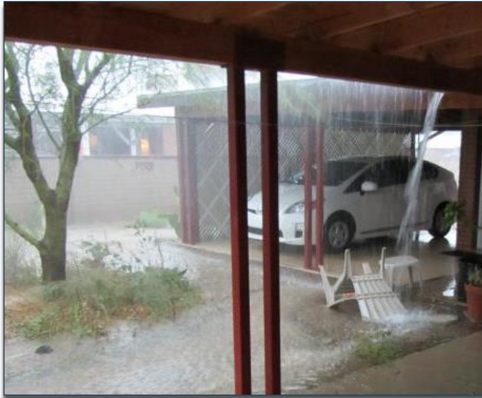
Photograph 3-2 Waterfall created by concentrated flows from two rooflines.
