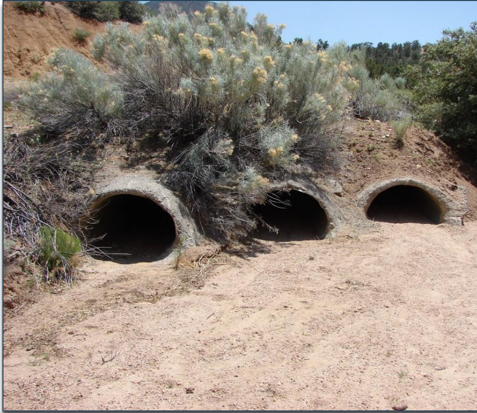
Photograph 3-4. Road culverts with reduced capacity due to sedimentation.
