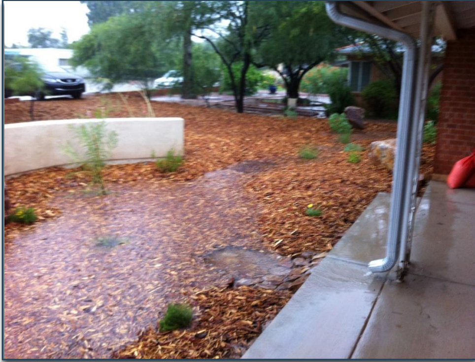
Photograph 7-6 The rain gardens in action providing an irrigation benefit while protecting the residential structure. Photo courtesy of Watershed Management Group.
