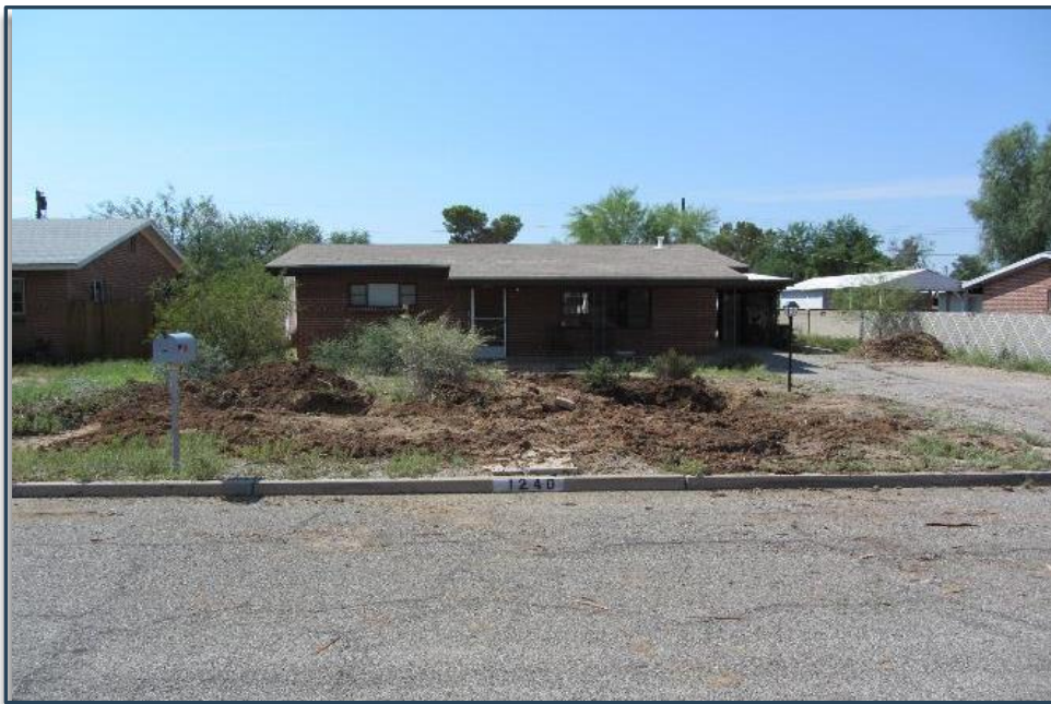
Photograph 7-10 The first step in the LID retrofit was to remove all non-native vegetation in order to improve shade, reduce water consumption, and increase soil infiltration rates.
