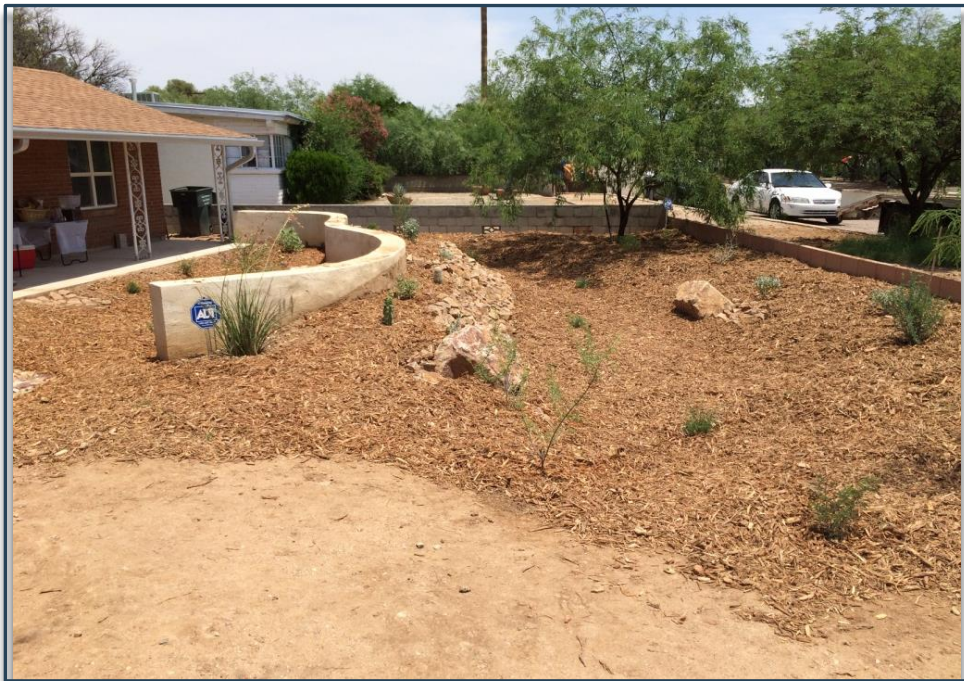
Photograph 7-5 After LID retrofit, the yard was lowered to provide drainage and retention capacity away from the home foundation. Photo courtesy of Watershed Management Group.
