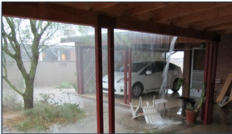
Photograph 7-8. Concentrated roof runoff creates a waterfall that ponds adjacent to the porch and drains toward the home's foundation.
