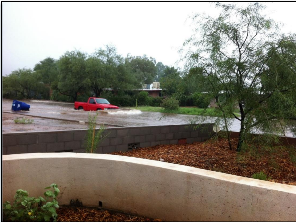
Photograph 7-3 Stormwater overtopping the curb does not flood the adjacent homes after project. Photo courtesy of Watershed Management Group.
