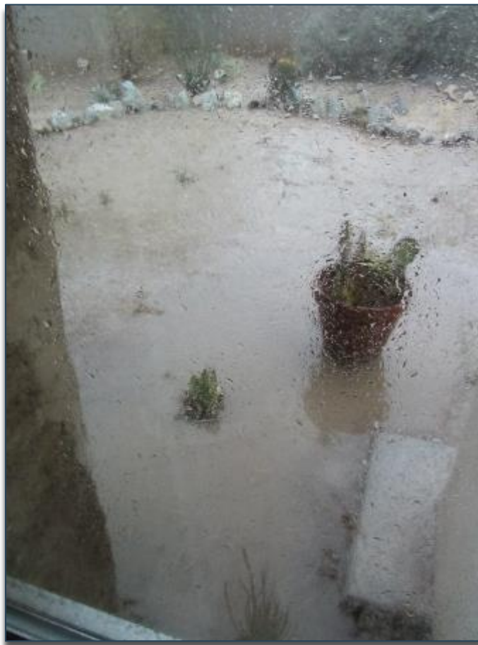
Photograph 3-3 Ponding adjacent to a home foundation and rammed earth wall.
