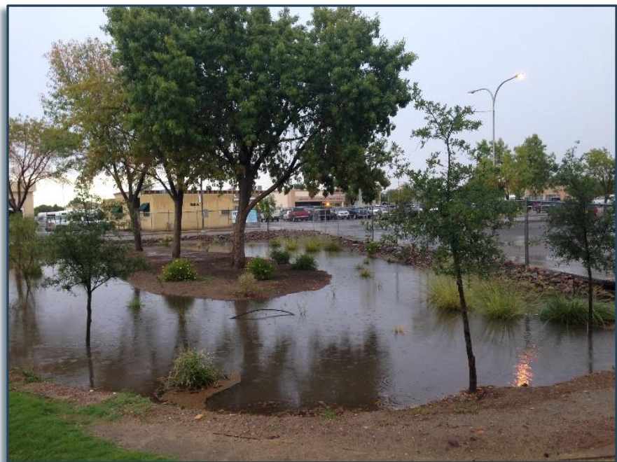
Photograph 2-1 Rain garden harvesting parking lot runoff for native grasses and trees in the City of Las Cruces, NM.
