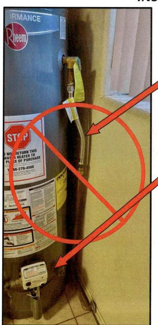
TEMPERATURE PRESSURE RELIEF VALVE IS REQUIRED TO BE HARD PLUMBED TO A DRIP PAN OR TO THE EXTERIOR TO PREVENT SCALDING AND/OR DAMAGE
