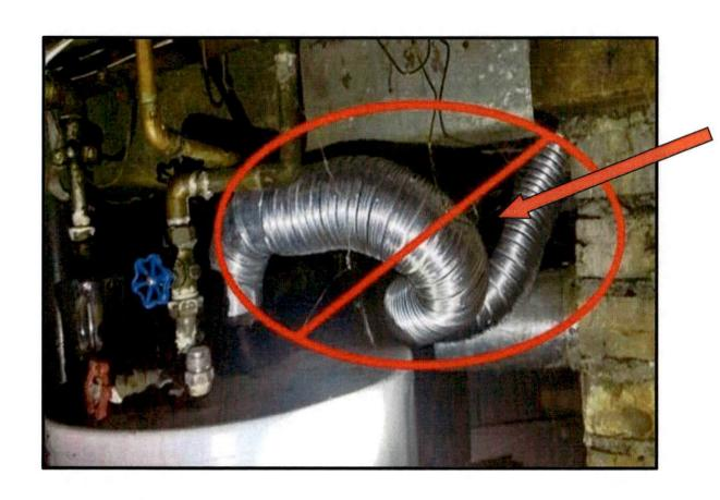
METAL DUCTING NOT RATED FOR HOT WATER HEATER, VENT MUST HAVE VERTICAL RISE FOR GRAVITY VENTING TO PREVENT BACK FEEDING OF GASES INTO THE ROOM
